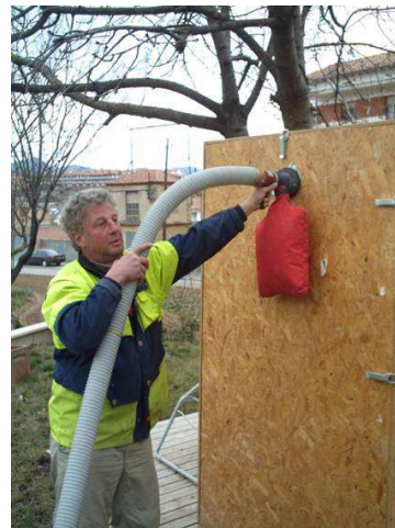
Cellulose projected: 0,040 W/m·K (newspaper, 10% Borax for fire resistance and as fungicide)
