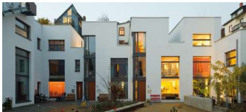
Residential building complex Passivhaus, 2009, Frankfurt, Arq. Rook
